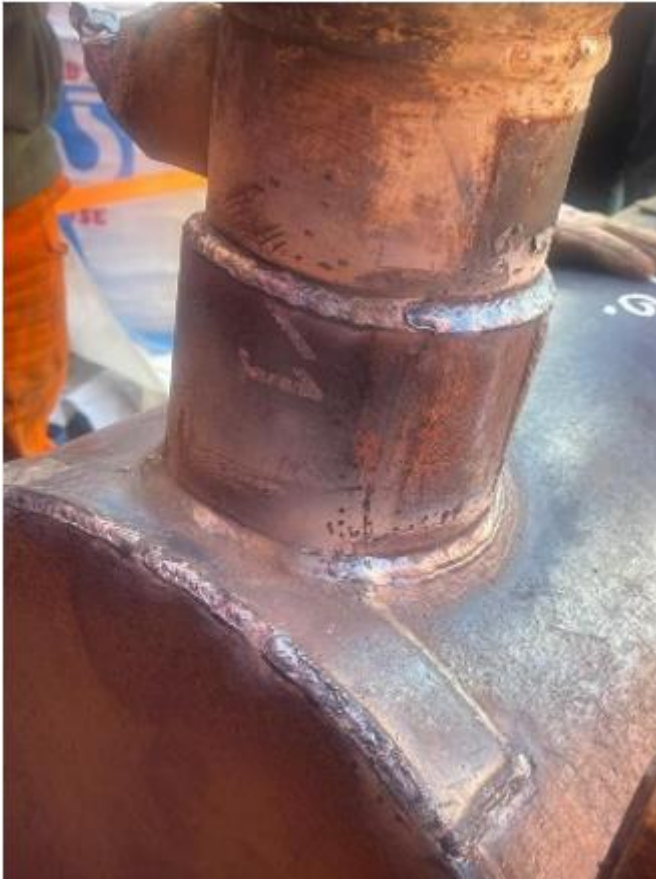
Sleeve welded at the area of corrosion
